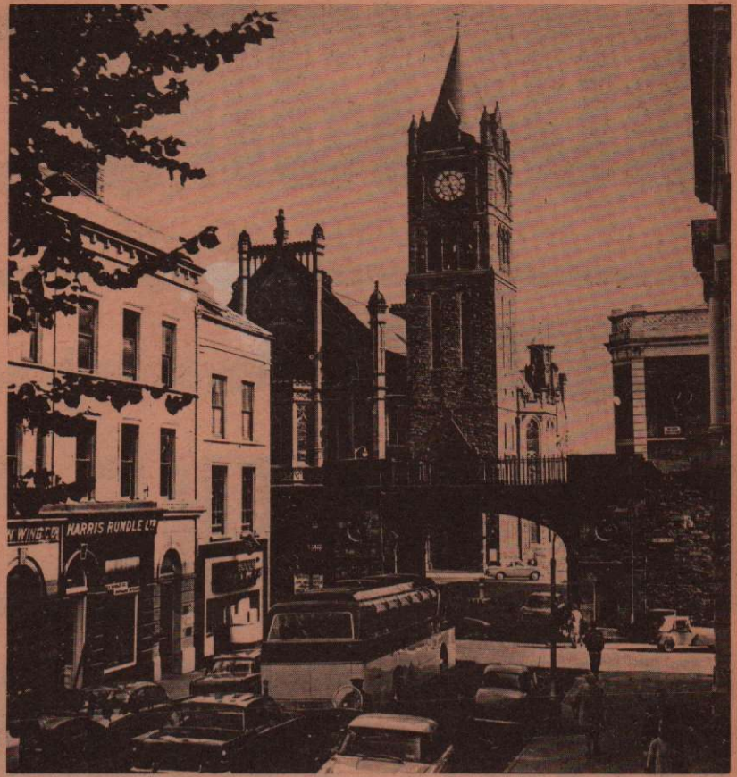
Derry's Guildhall - seat of Gerrymandered power
