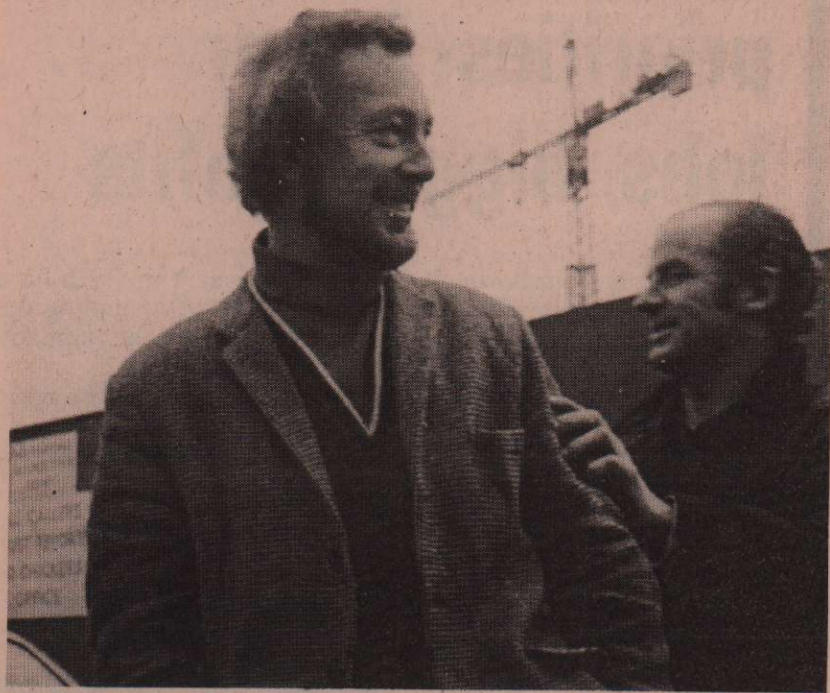
Owen McSweeney (right), carpenters' steward at the World's End site, and John Fontaine, strike committee treasurer, outside the site last week.
